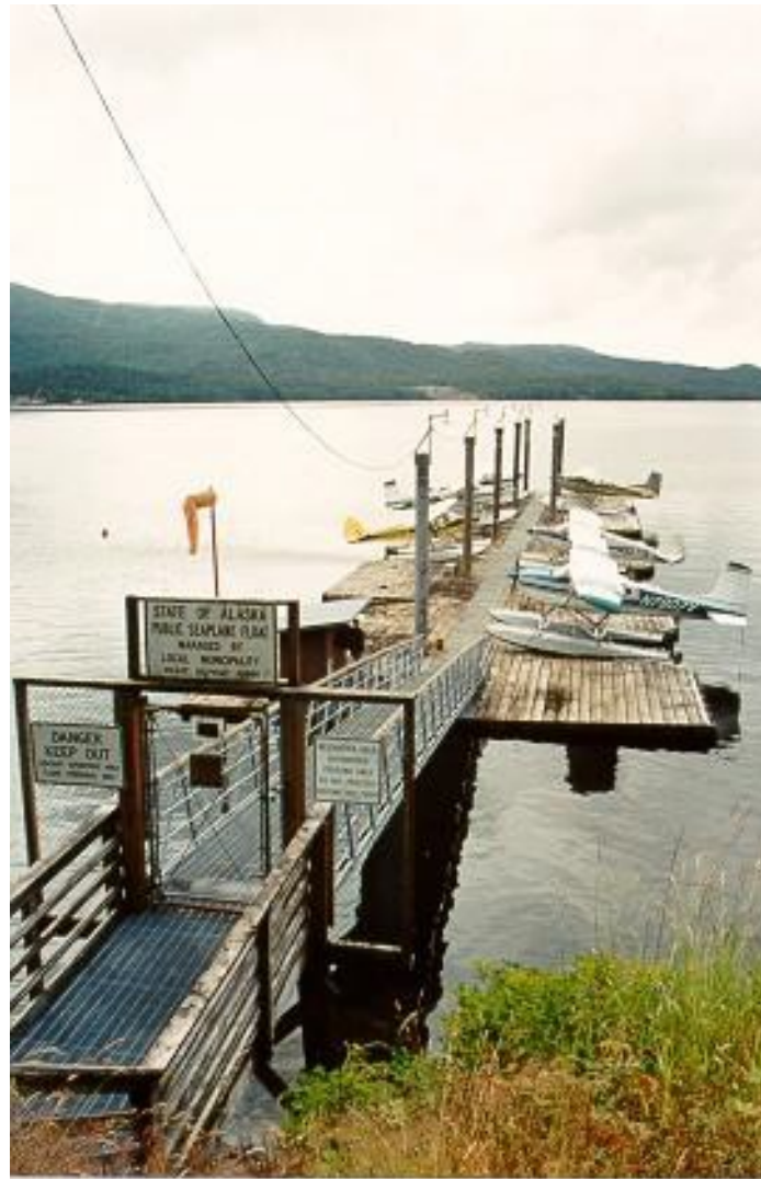
Figure 2-7. Example of a gangway in Alaska
